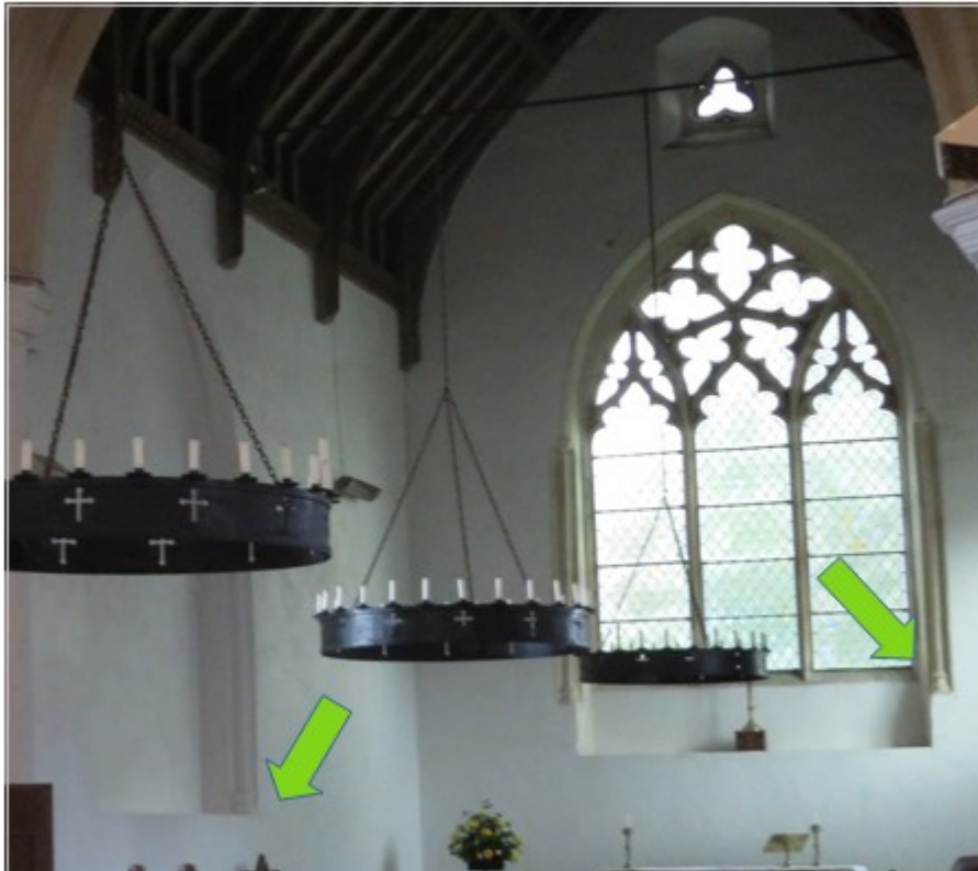
Figure 17 showing the chancel window mouldings
