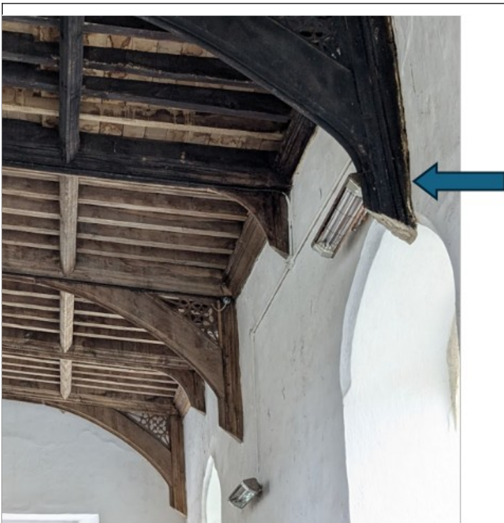
Figure 29 South Aisle roof structure
