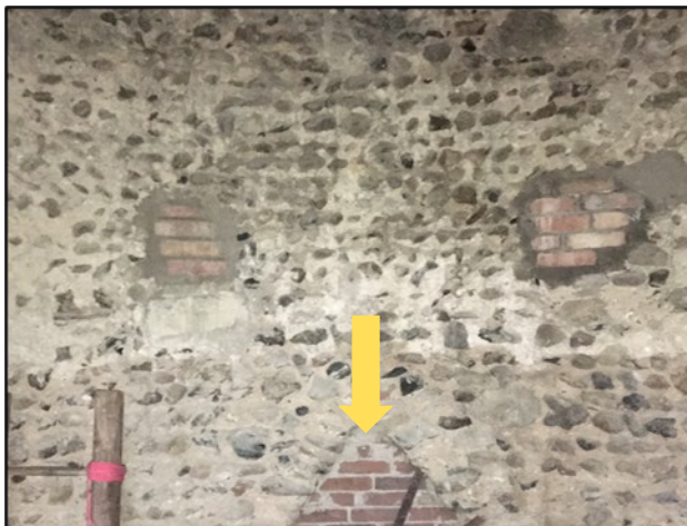
Figure 3 inside of tower showing filled areas
